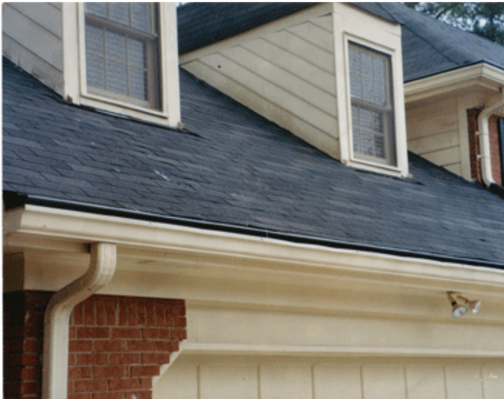
The same house after getting gutter protection.
